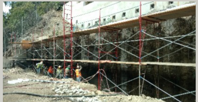
Vapor Lock - Hillside Pinning with NO Fly Ash; Beverly Hills, CA
