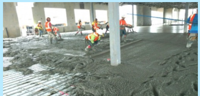
Second Floor Vapor Lock Moisture/Vapor Control Integral Concrete placement - Warranted & Insured protection - all critical paths met.
